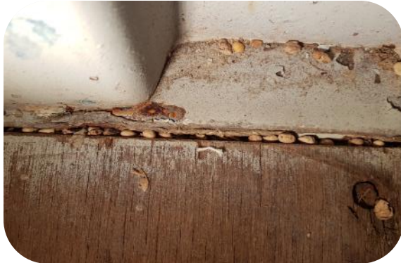
Gaps between floorboard and container wall
